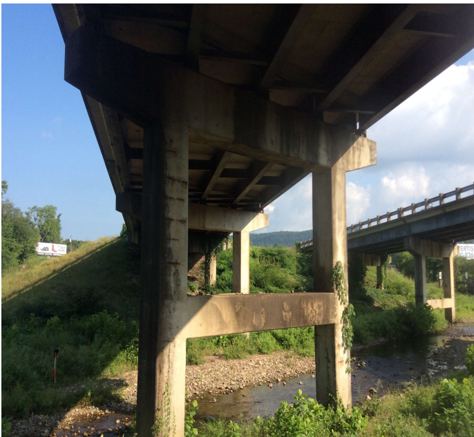
PHOTO 1 Description Bent 4, ahead side, exposed rebar on columns.
